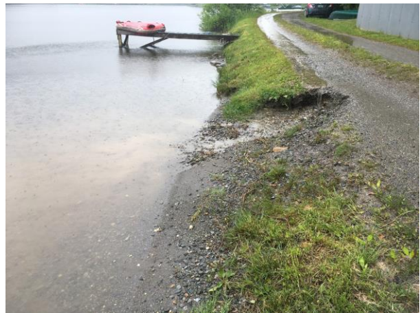
Figure 4: A culvert on the Gihon River with poor channel alignment had the lowest problem area score (left photo, Project SC-3). Erosion and transport of sediment from Lake Shore Road directly to the Lake was the highest problem area score (right photo, Project SW-11).
